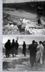
The area of Zichen-Zussen-Bolder is undermined by a dense network of cavities. These cavities were excavated in Cretaceous sediments since Roman times for marl that was used as construction material. After the second World War the caves were used for mushroom growing. In order to let in large lorries the tunnels were enlarged. On December 23th 1958 a real disaster happened when 4 ha collapsed, causing the death of 18 people.
